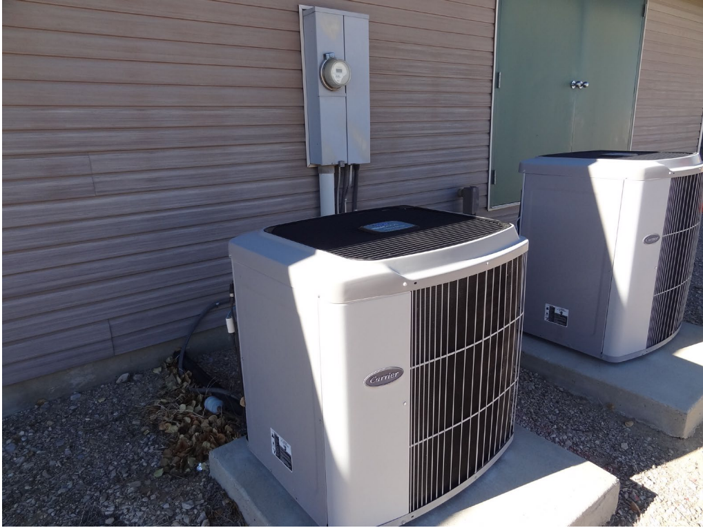
Ely Wildlife Field Office - Building #2127 Description: HVAC R-22 Equipment Replacement Needed.
