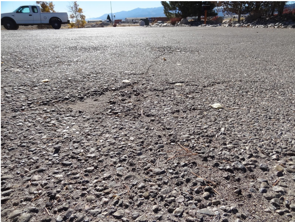
Ely Wildlife Field Office Site - Site #9825 Description: AC Paving Crack Fill & Seal.
